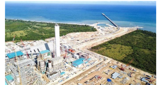
Punta Catalina - Coal-Fired Power Plant - Spina Group
